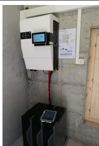
Figure 3 : Studer-Innotec Next3 inverter (FMA)
